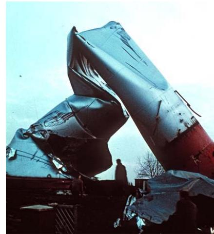
Buckled & collapsed cylindrical shell water tower
