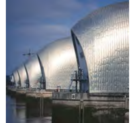
Above The Thames Barrier, River Thames, London.
