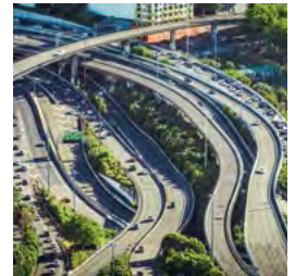
Above High angle view of traffic on a complex series of roads and intersections in Auckland, New Zealand.
