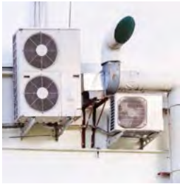
Above Air conditioning compressors.
