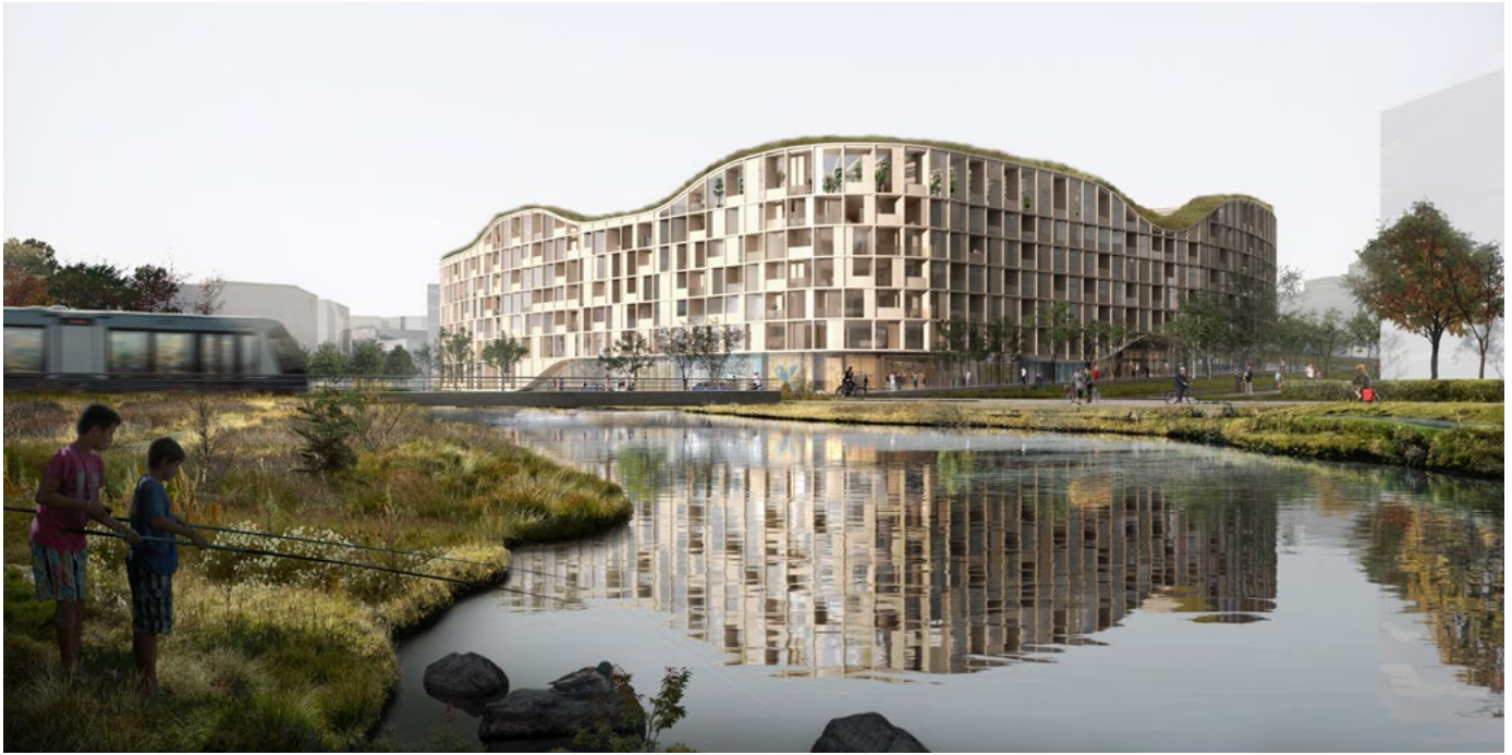
Image: Designed by Jakob+MacFarlane architects, Living Landscape is a mixed-use building set in a former landfill site in Reykjavik. Making use of a prefabricated cross-laminated timber structure will reduce the building's embodied carbon footprint by almost 80% compared to a typical concrete building, while operational emissions are minimised through an integrated waste-heat recovery system, comprehensive insulation and a renewable energy supply. © Jakob+MacFarlane.
